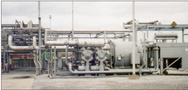
Figure 4.13 – “Pipeline” BOG Compressor.
